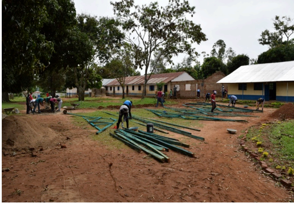
Above: Day 1 on the work site
