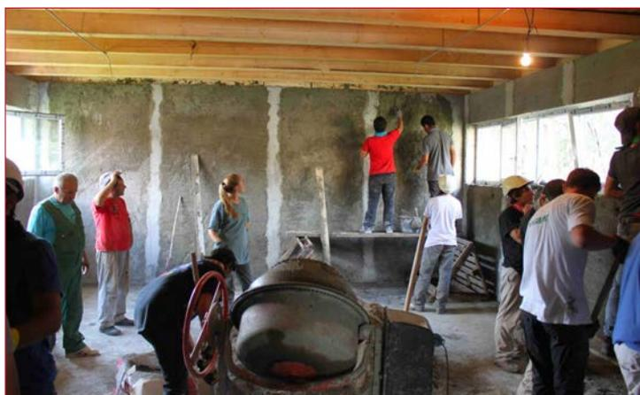
The team continued to work hard in the final phase of the project work at the youth/community centre, plastering the walls with first rough cement and then fine smooth cement and finally buffered it so it was completely ready for painting. They also managed to fit in painting and staining the stage at the major's office which is used for town events and everyone got a certificate of excellence from the major!
